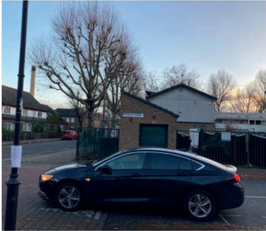
1 Looking south towards existing buildings on site
