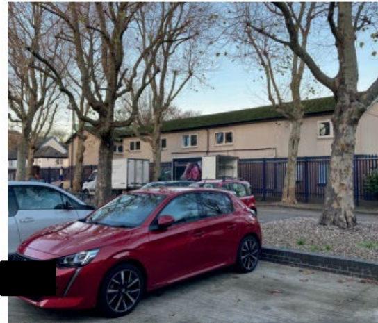
4 Looking northeast towards the existing buildings on site
