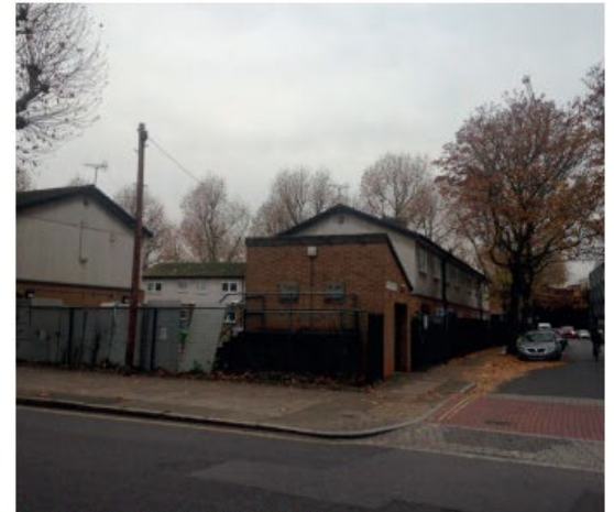
6 Looking west towards existing buildings on site
