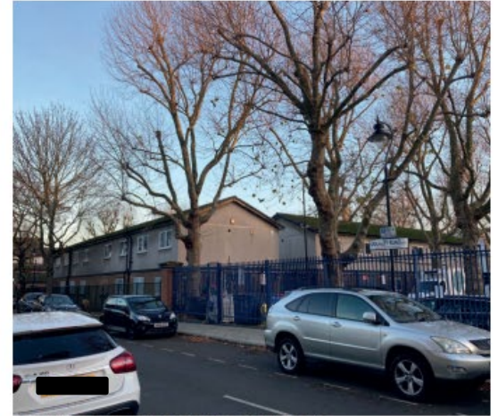
3 Looking southeast towards the existing buildings on site
